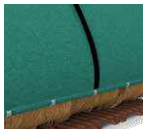
C. Overlap FLOREX® 160 for 20 cm and join with hook and loop tape.
